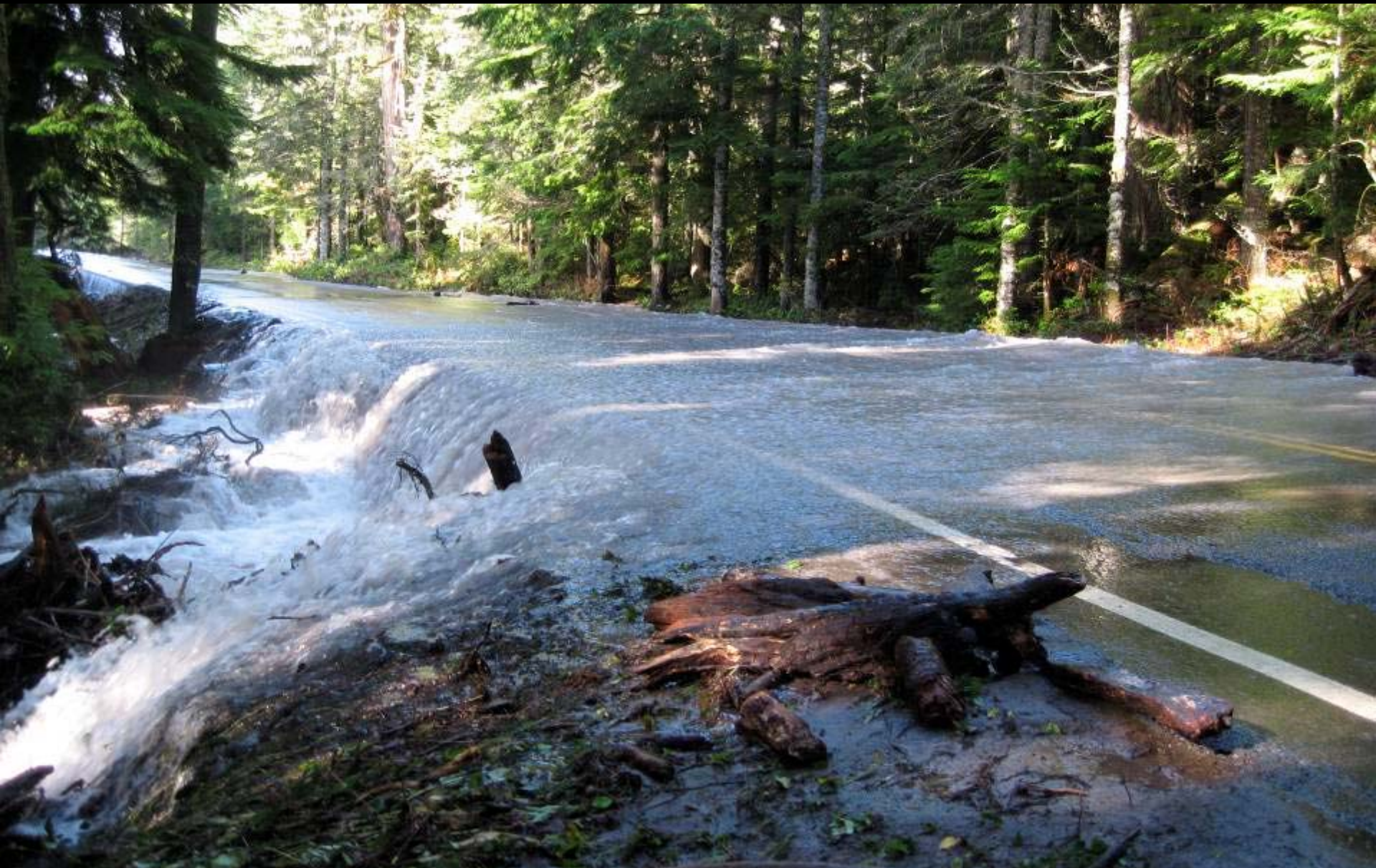
Kautz Creek flowing across the road east of the bridge
