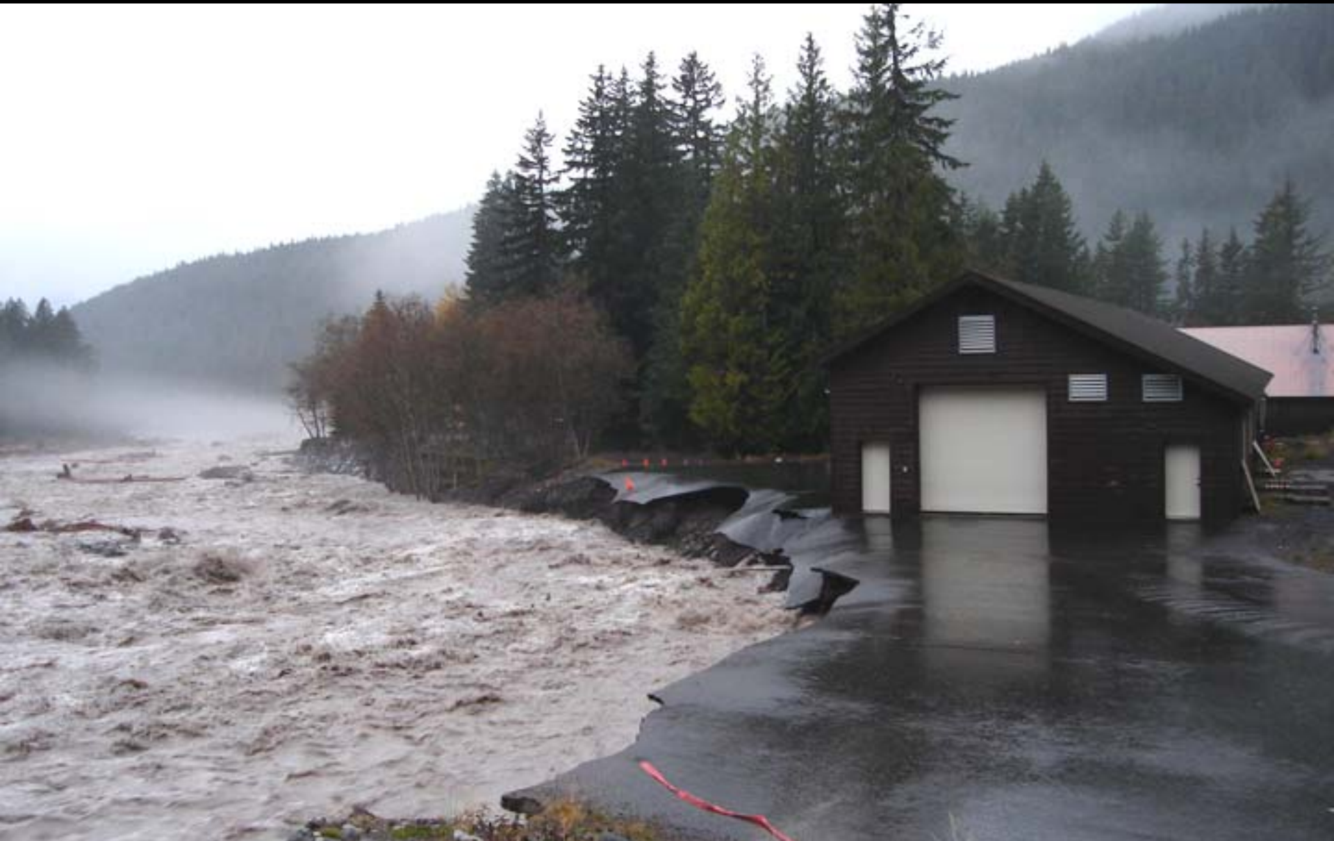
The Emergency Operations Center at Longmire, during the flood
