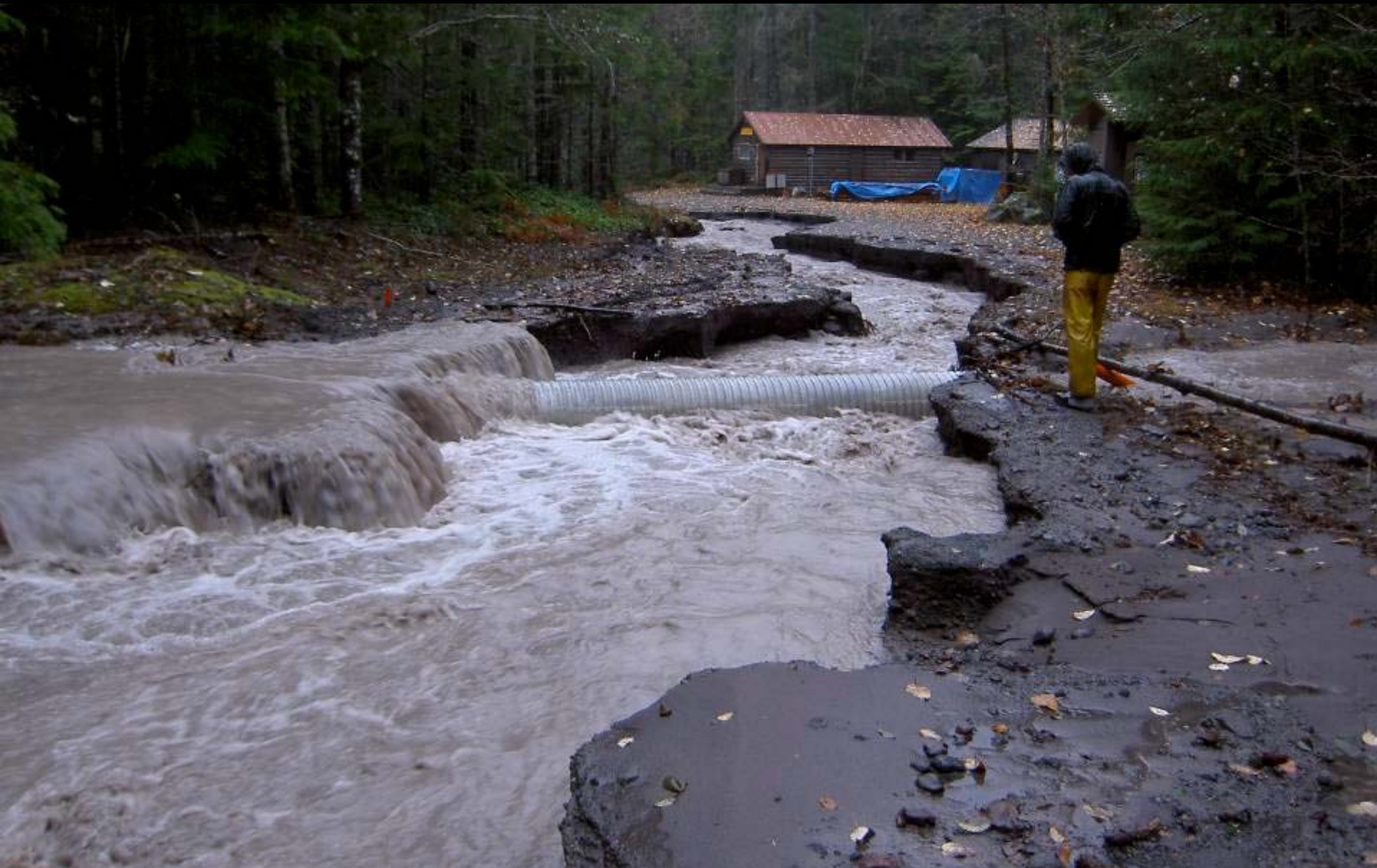
The new creek channel flows through the middle of the Kautz Helibase
