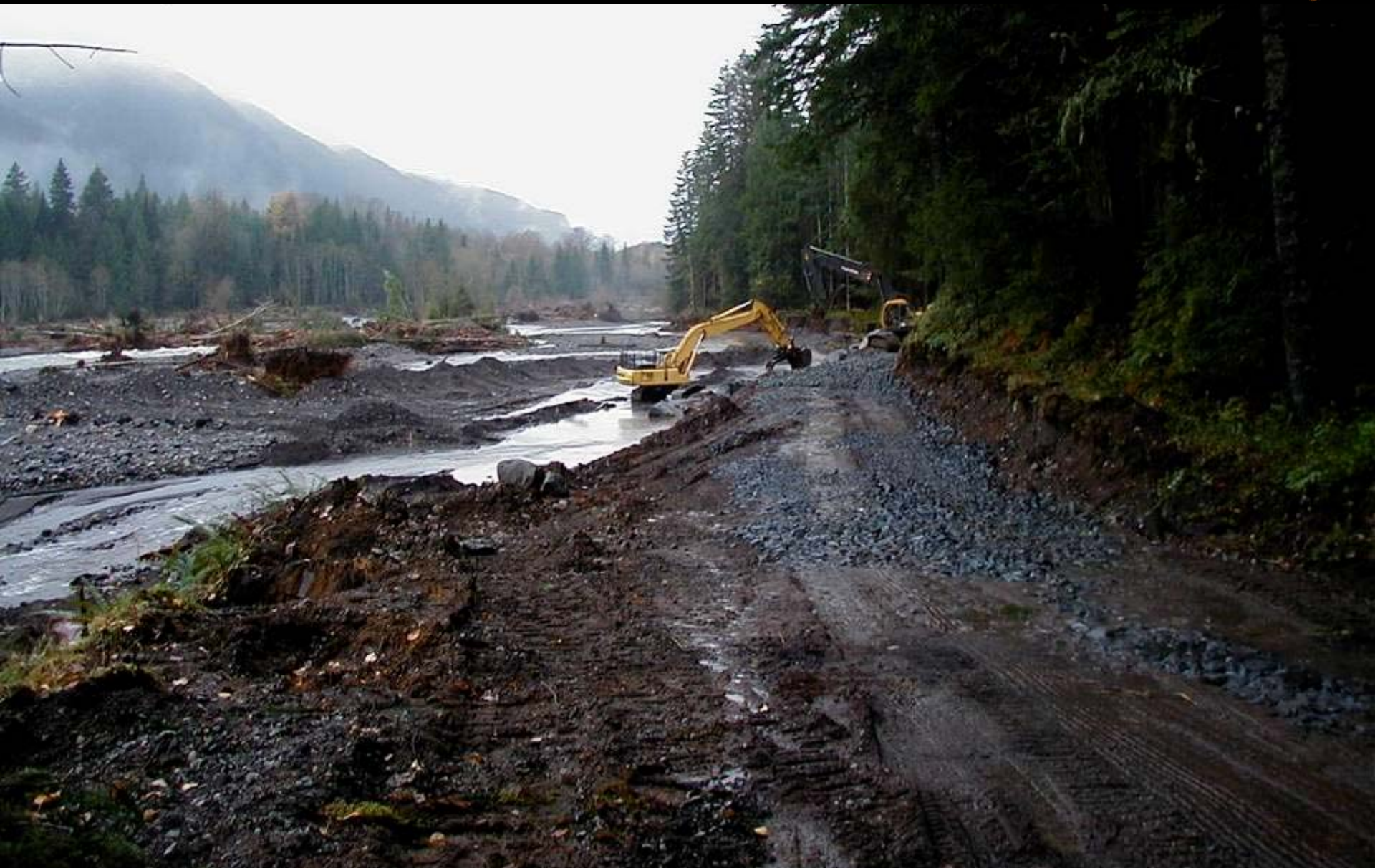
Rebuilding the Nisqually Road
