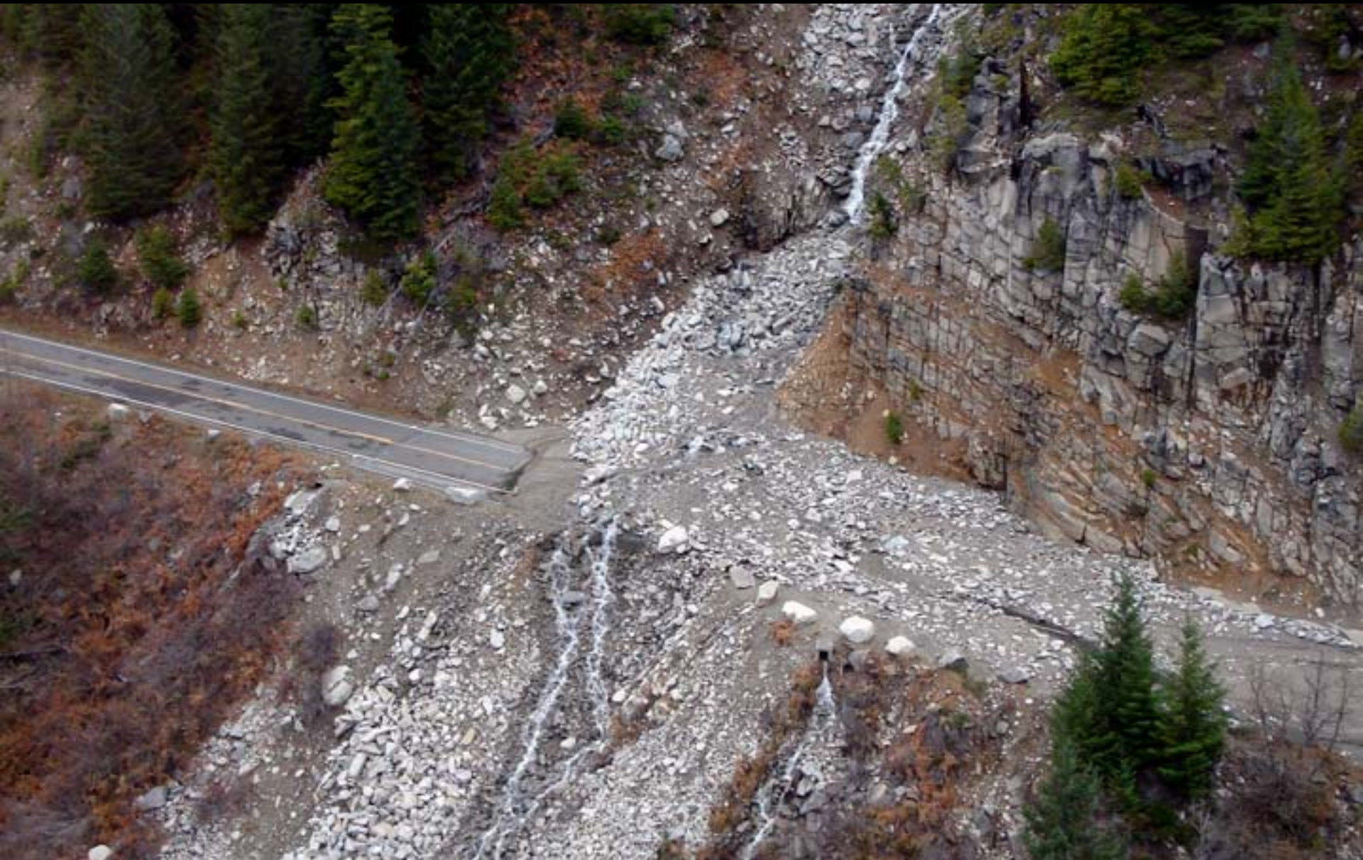
Landslide below Stevens Ridge in Stevens Canyon
