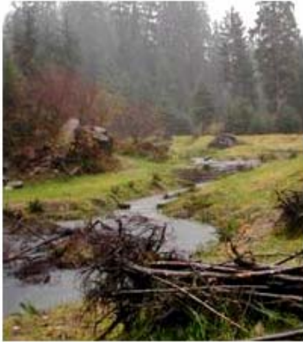
Floodplain channel dug
