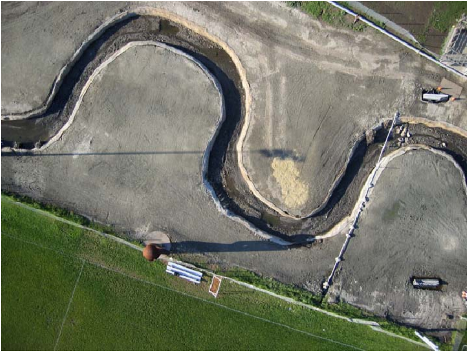
Restored reach formerly in a straight culvert, Berkeley, CA
